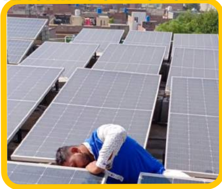
190kW Grid Tie Solar
